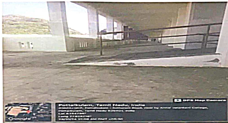
RAMP IN MECHANICAL BLOCK
