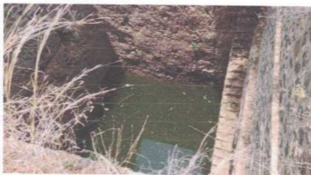
Figure. 6.1: Rain water harvesting well
