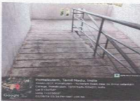
RAMP IN MECHANICAL BLOCK
