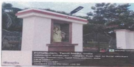
Solar street light in main gate
