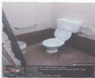
Disabled friendly washroom
